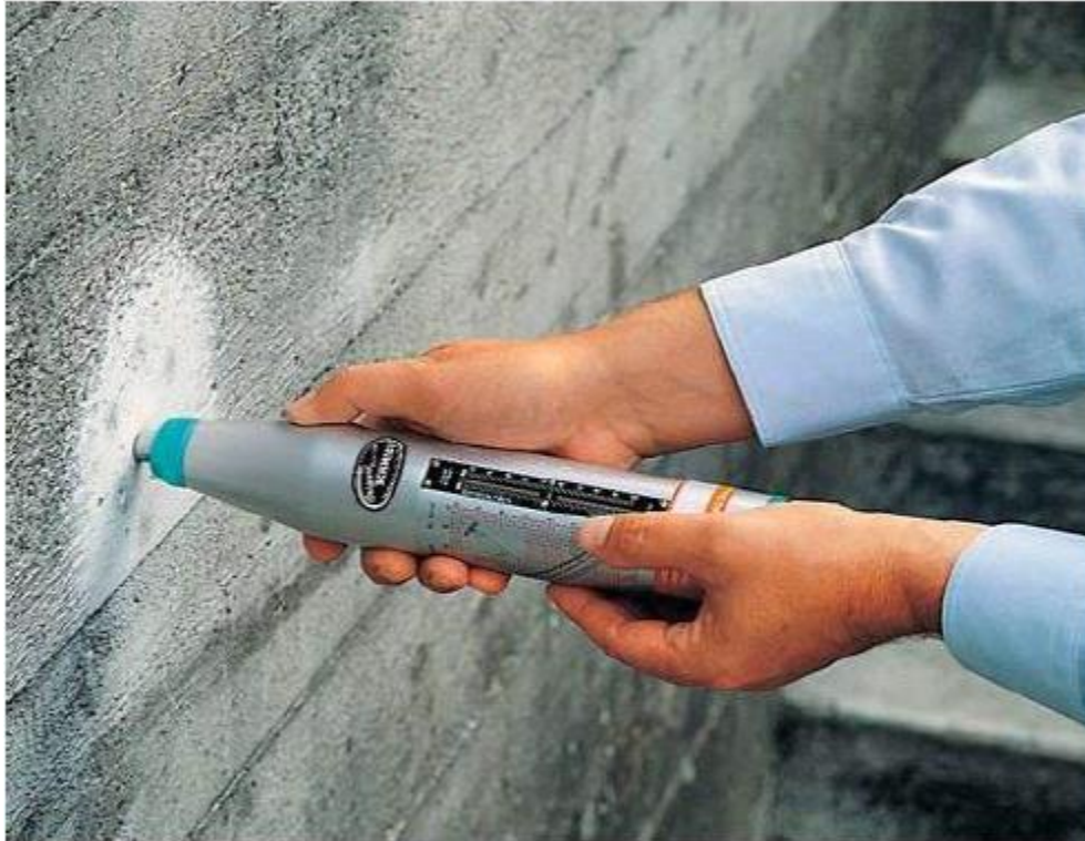
NDT test on concrete
