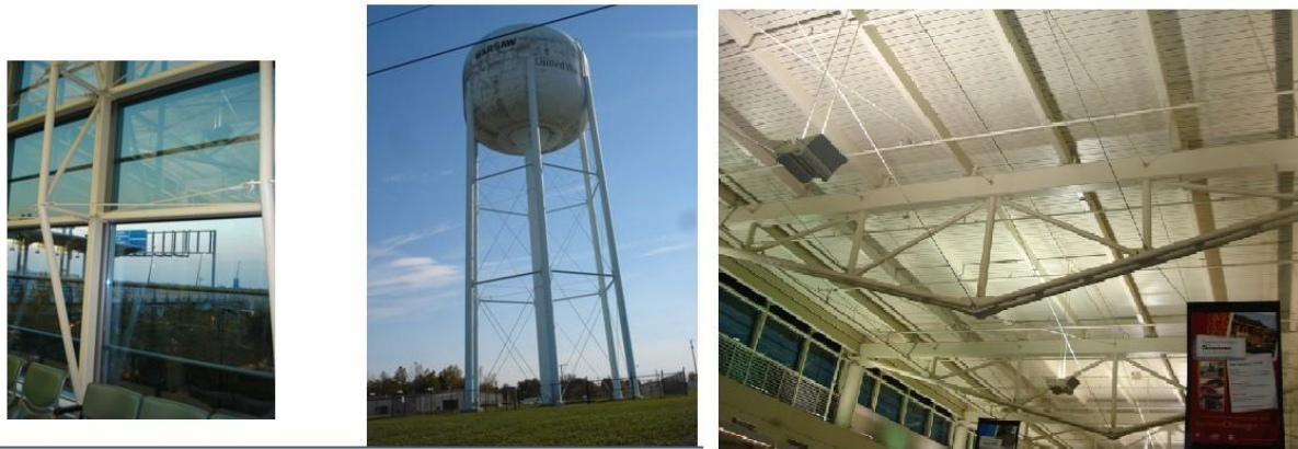
Tie Rods in Structures
