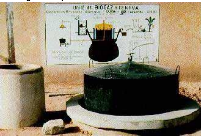
Figure 7: Floating-drum plant in Mauretania
